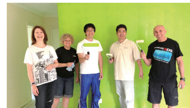
Employee volunteers repainting walls of a hospice room
